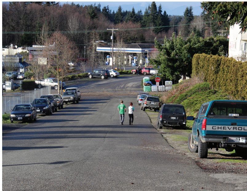
above: existing condition
