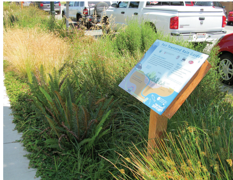
above: bioretention swale
