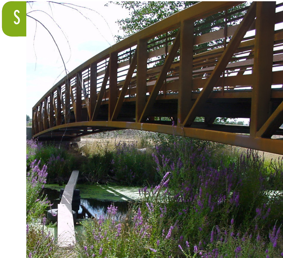
Figure 3S: Typical Steel Bridge
