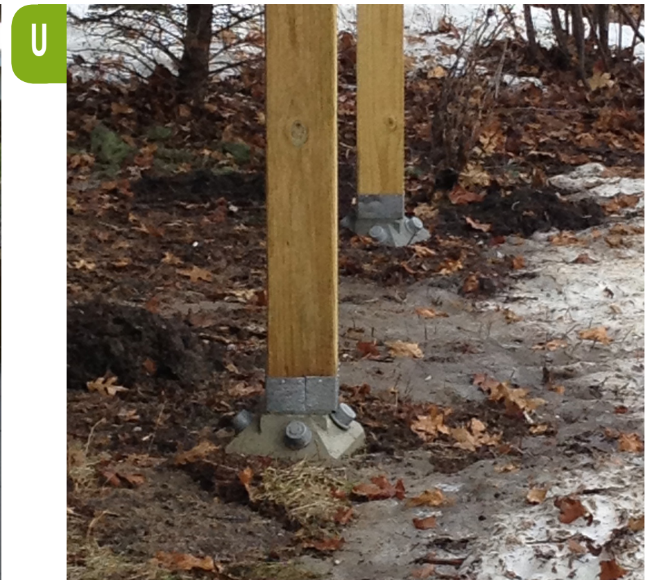
Figure 3U: Pin Pile Footings (Image Courtesy of Diamond Pier)
