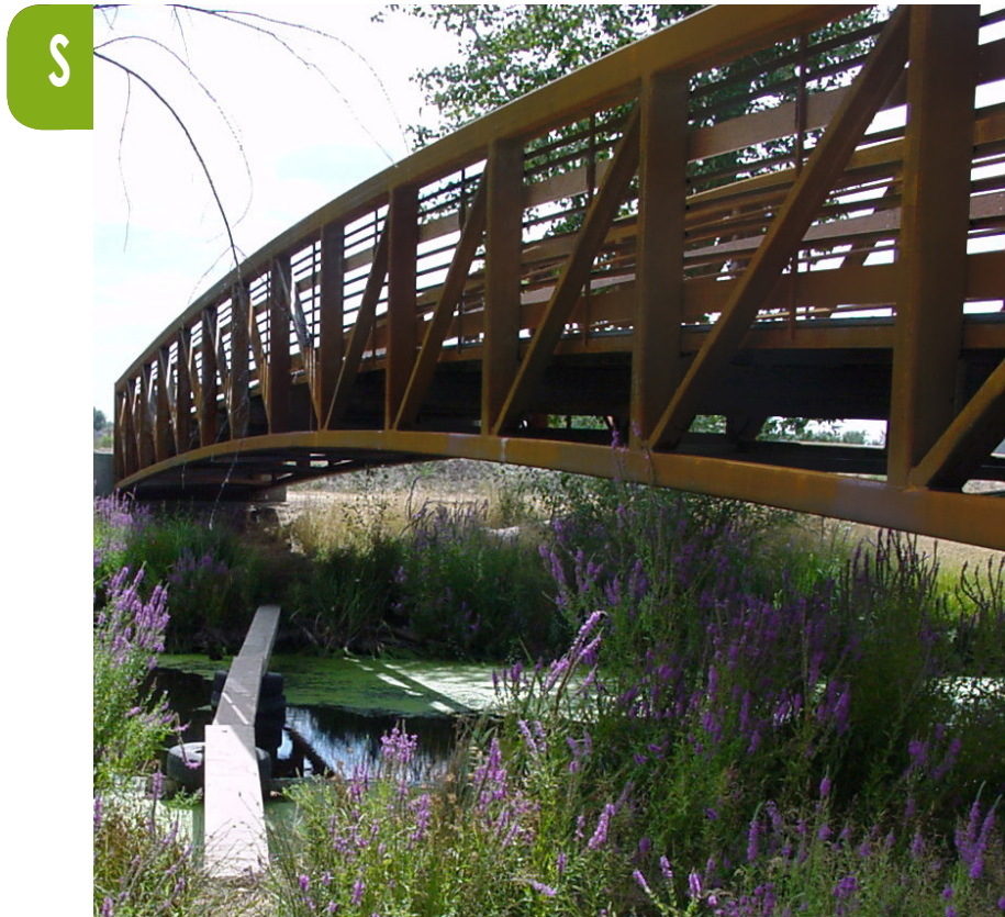
Figure 3S: Typical Steel Bridge
